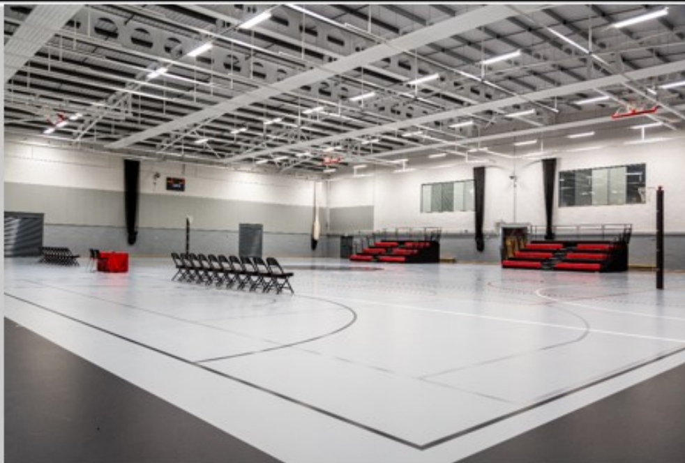
Seamless polyurethane over a sprung base at Hartpury College & University
